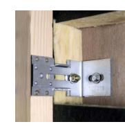
The adjustable brackets are alternately placed to the left and the right of the vertical batten. This helps to prevent the batten twisting and keeps a straight supporting frame.
